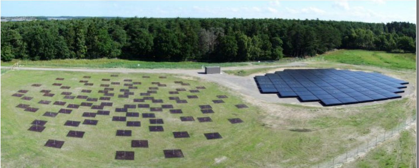
Figure 11: The LOFAR station at Chalmers, Sweden: an example of how a modern telescope can take the form of a sensor array (brown, low-frequency tiles on the left; grey, high frequency pads on the right), and also how a Dutch initiative is spreading over all of Europe, linked by high-speed fibres for communication. Credit: ASTRON
