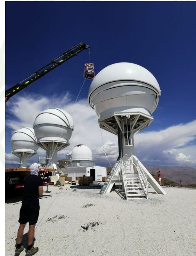
Third telescope being installed (Jan 2020)
