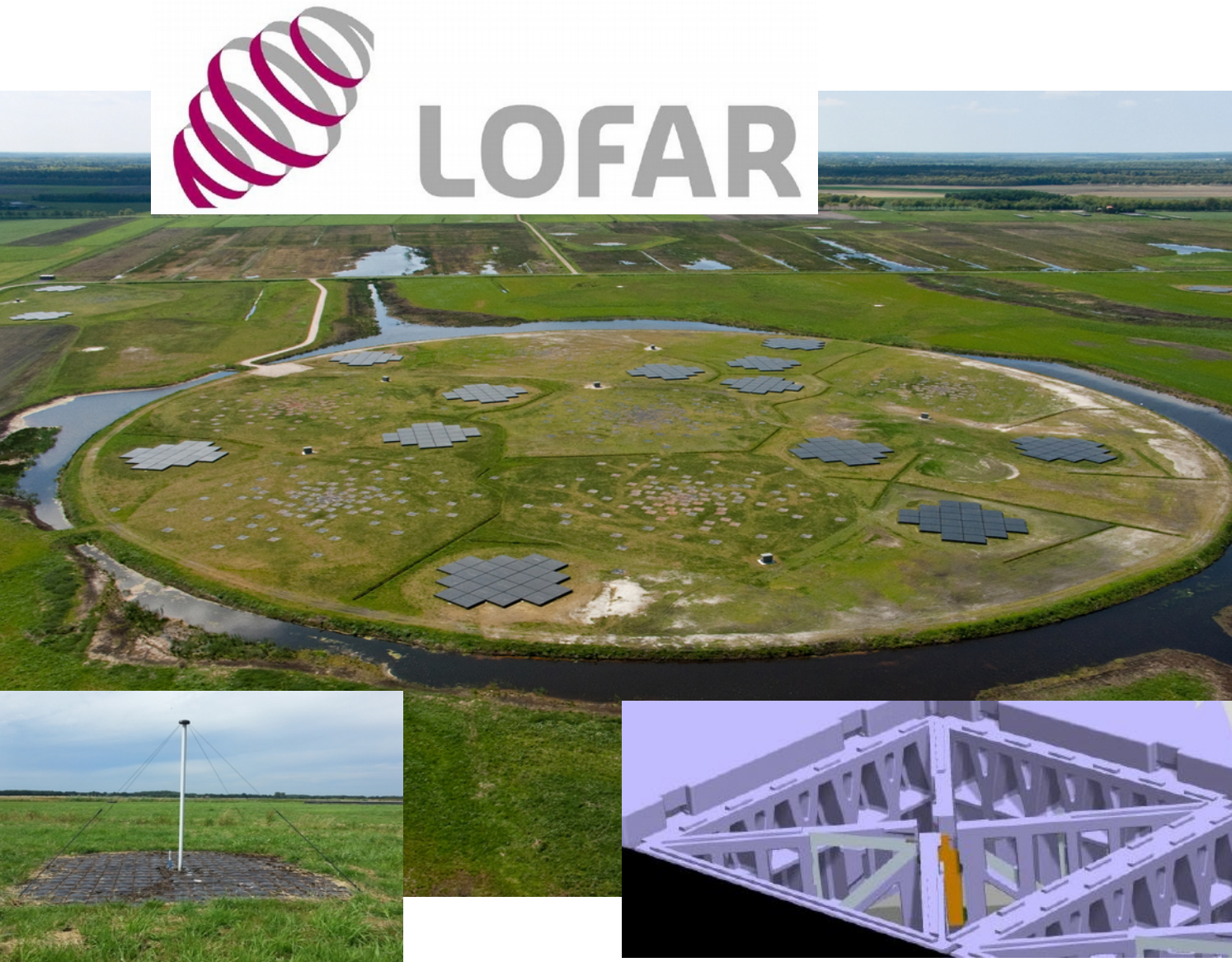
Top: LOW Frequency Array (LOFAR) in Exloo, Drenthe Province. Bottom: picture of one Low Band Antenna 30 - 80 MHz (left), and High Band Antenna 110 - 240 MHz (right)
