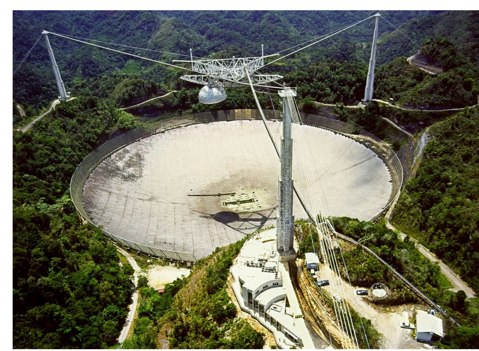
ARECIBO radio telescope in Arecibo, Puerto Rico - single-dish telescope with a diameter of 305 meters; observing frequencies: 8 MHz, 47 MHz, 430 MHz and 2.38 GHz
