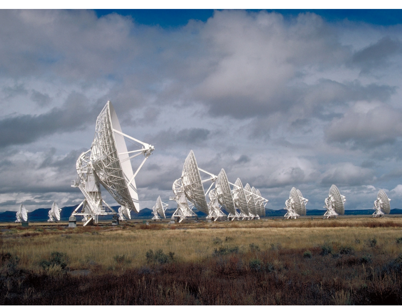
Very Large Array in New Mexico; 27 radio antennas with a diameter of 25 meters; the combination of all antennas reaches a sensitivity of an equivalent 130 meters diameter single-dish
