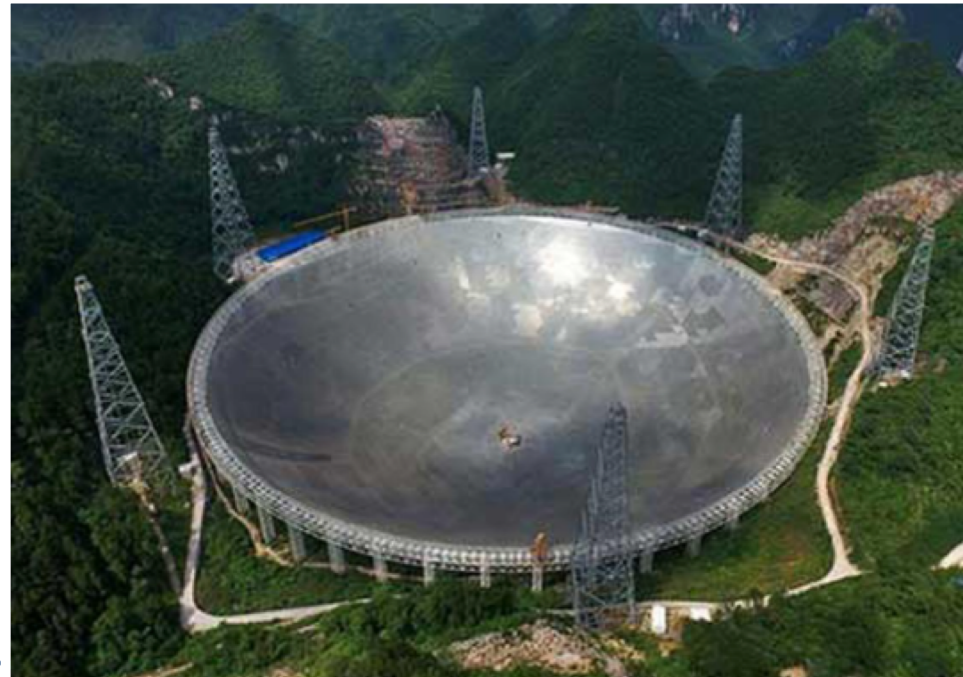
FAST, China diameter: 500 m Resolutie ( \lambda 21\text{cm} ) \theta = 0,02^\circ
