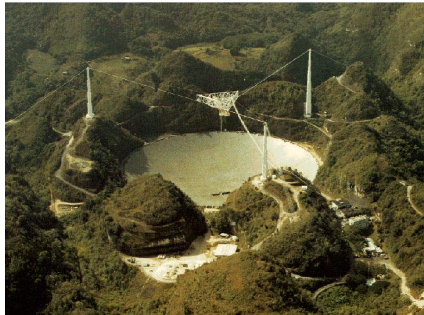
Arecibo, Puerto Rico diameter: 305 m Resolutie ( \lambda 21\text{cm} ) \theta = 0,04^\circ
